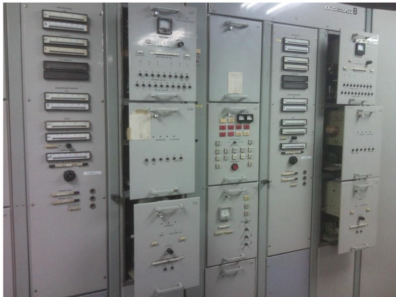
Figure 1: Front panel of the existing RF power system.
