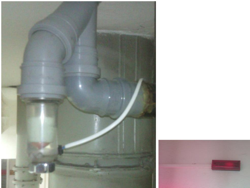
Figure 3: Water leakage sensor (left) and water leakage indicator lamp (right).
